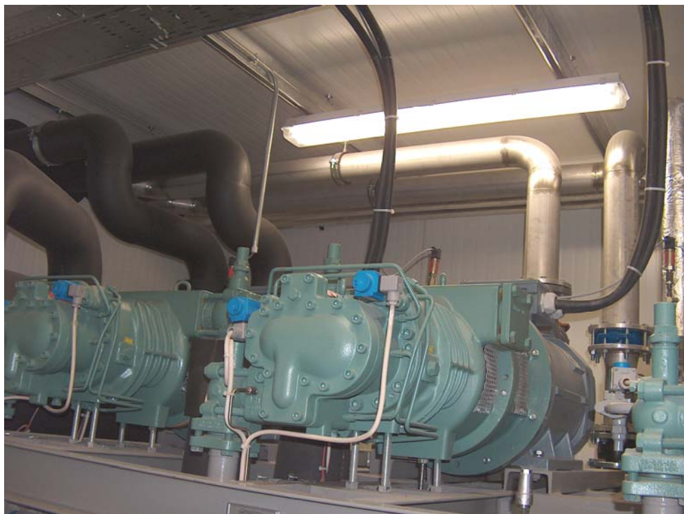
Rack com compressores Octagon (CO2)
