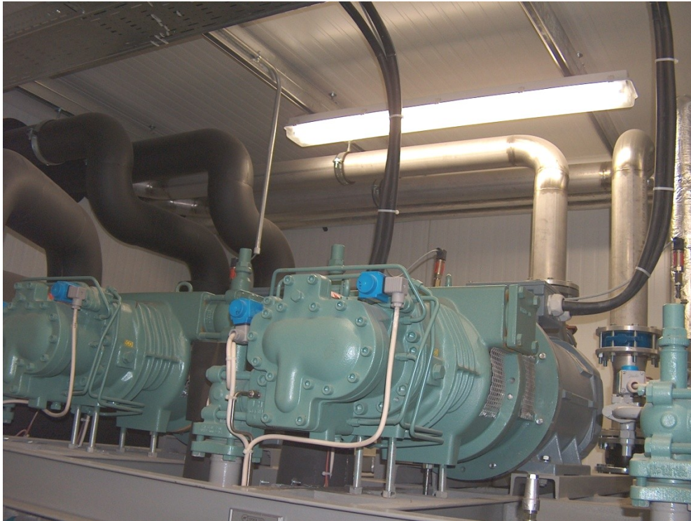
Rack com compressores Octagon (CO2)
